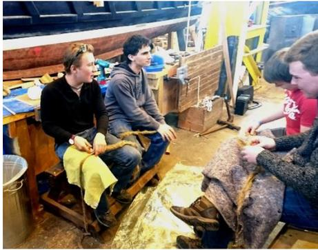
*Fig. 5: Spinning oakum for caulking.*
